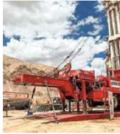
A view of ONGC's advanced drilling rig. File @LG_LADAKH X/ANI
